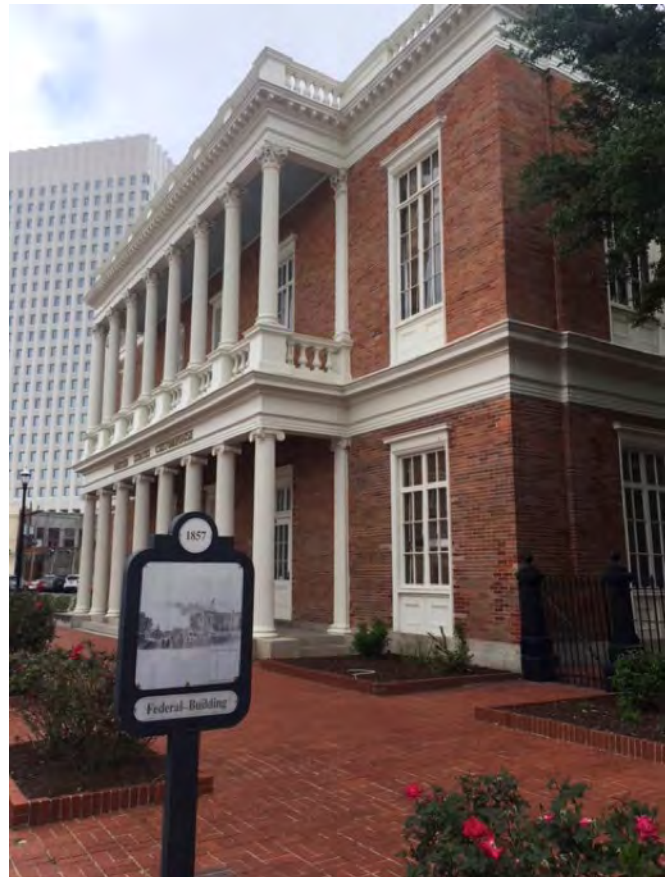
Judge Winch aspired to serve in the building preserved as Galveston’s Federal Customs House. Photo by David A. Furlow.
